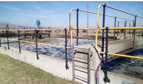
Refurbishment of sewer plant that was vandalised
