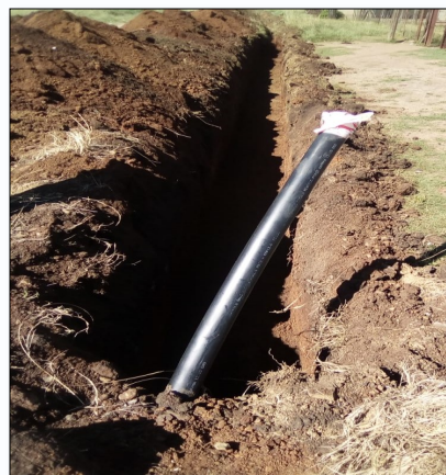
Installation of water pipelines that will separate sewer and water lines
