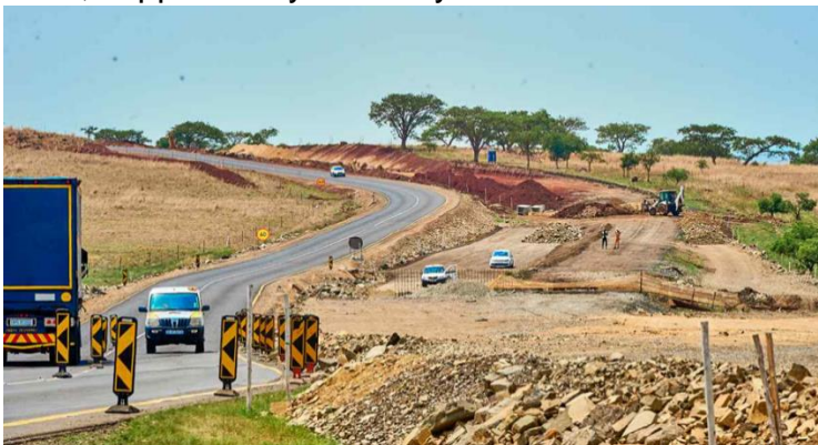
N11 ROAD CONSTRUCTION
